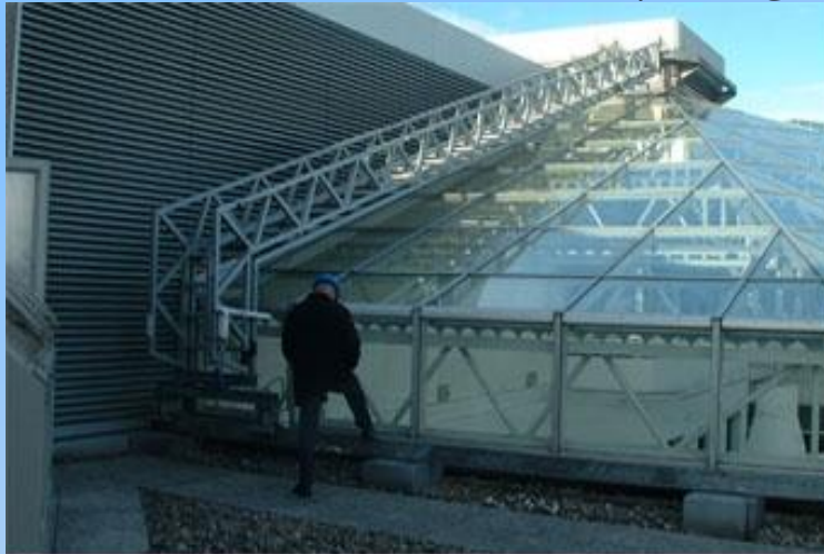
MOTORIZED TRAVELLING LADDER MATERIAL : ALUMINIUM LENGTH : 3 - 12 M WORKING HEIGHT : NO LIMIT
