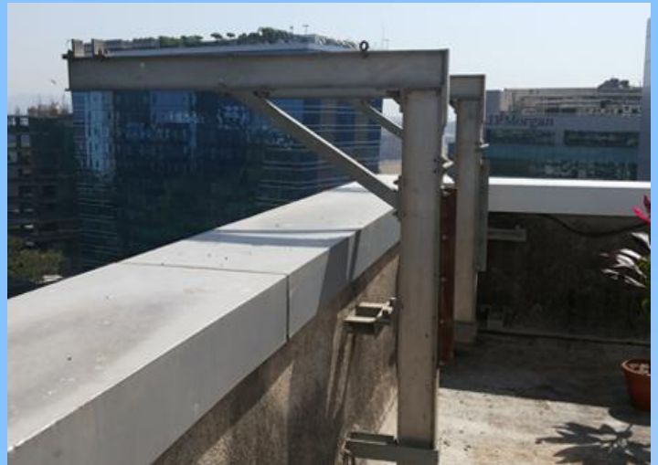
PARAPET MOUNTED DAVIT SYSTEM
